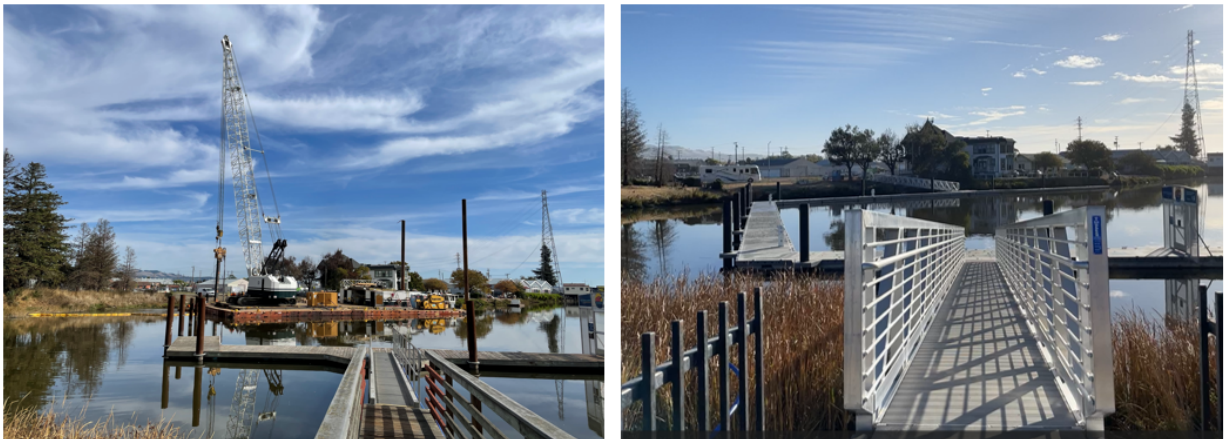
Figure 2: Mid-section docks and piles before (left) and after (right) with new utility pedestal
