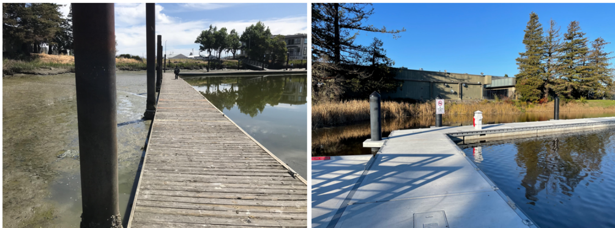
Figure 2: Mid-section docks and piles before (left) and after (right) with new utility pedestal
