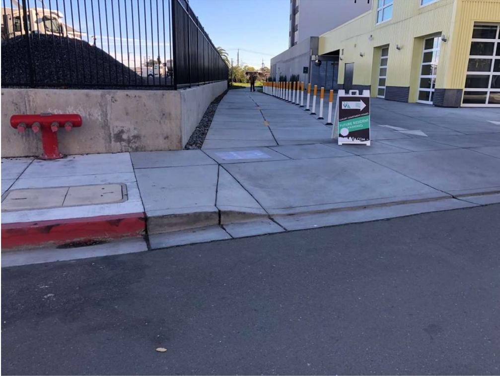
The curb cut doesn't match the bike path, so again, getting onto the path is tricky.
