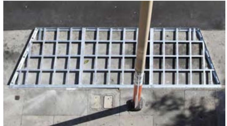
Figure 72. Installed steel sub-structure, "Peace Keeper" parklet, San Francisco, CA. Credit: Martha Traer
