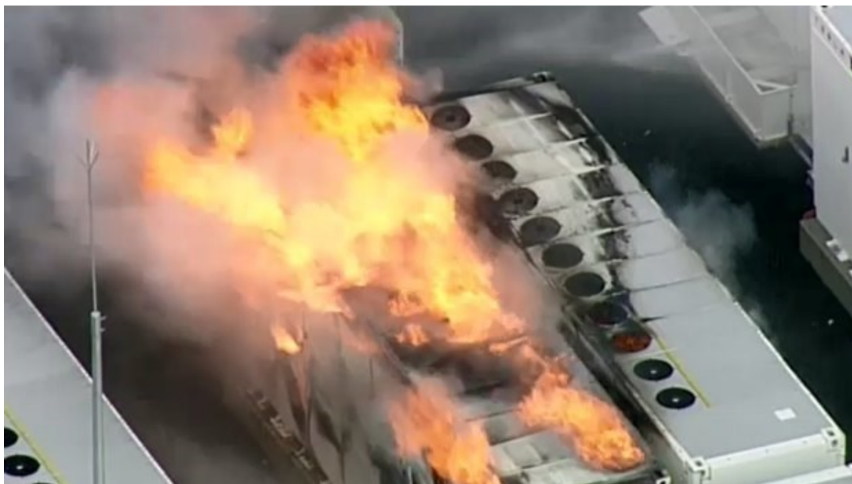
Figure 3. Containerized BESS After Thermal Runaway Initiates.
