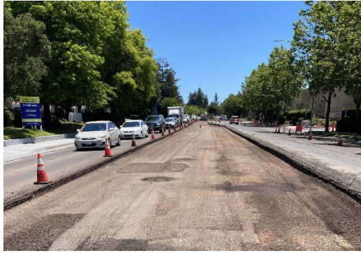
Step 1 Grinding (milling) existing road pavement
