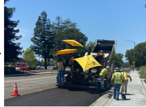
Step 3 Placement of recycled material as base layer
