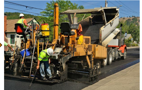
Step 4 Finish paving with new asphalt
