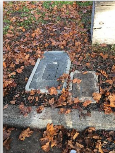
Residential Water Service Connection & Meter & Service Valve Boxes
