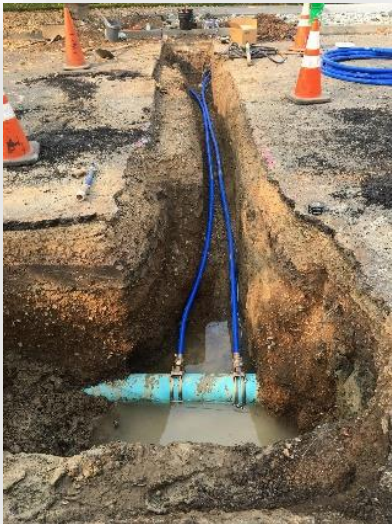
Residential Water Service Connection & Meter & Service Valve Boxes
