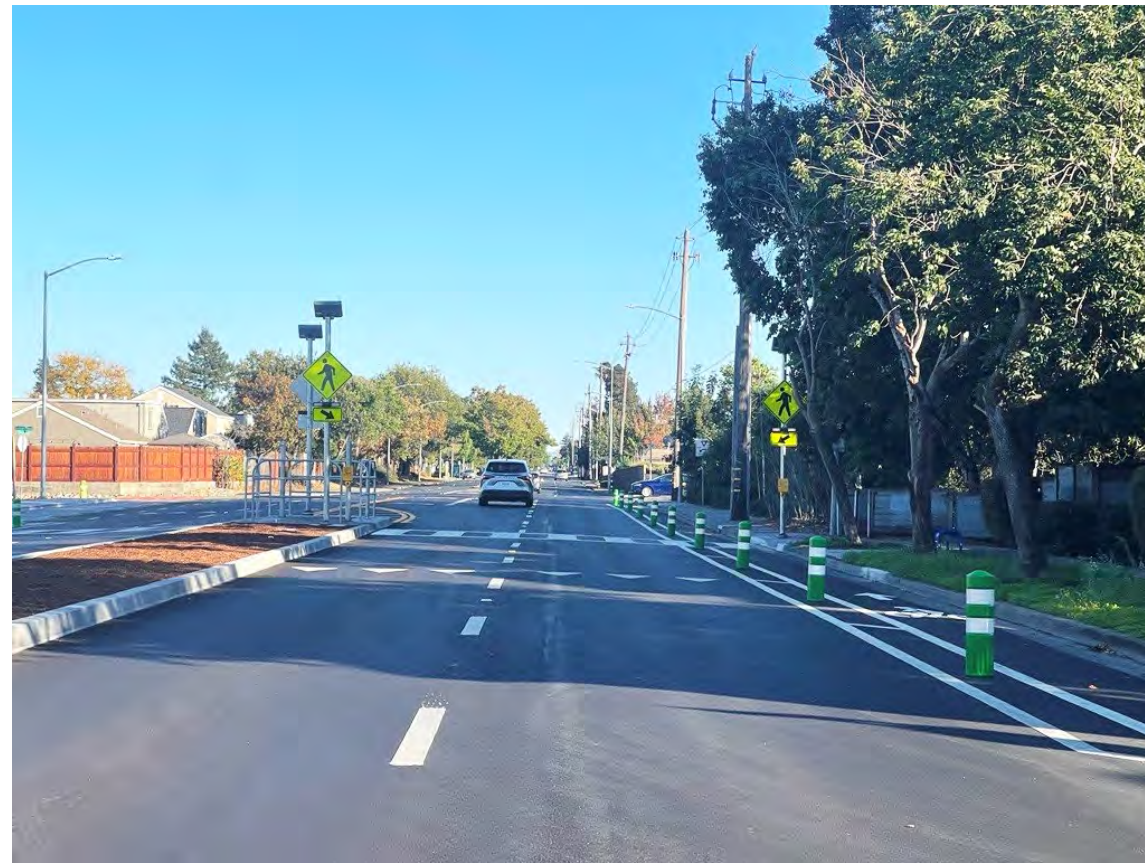
N. McDowell Blvd. Complete Streets Project - Before and After (K-71 pylons in the bike lane buffer zone)
