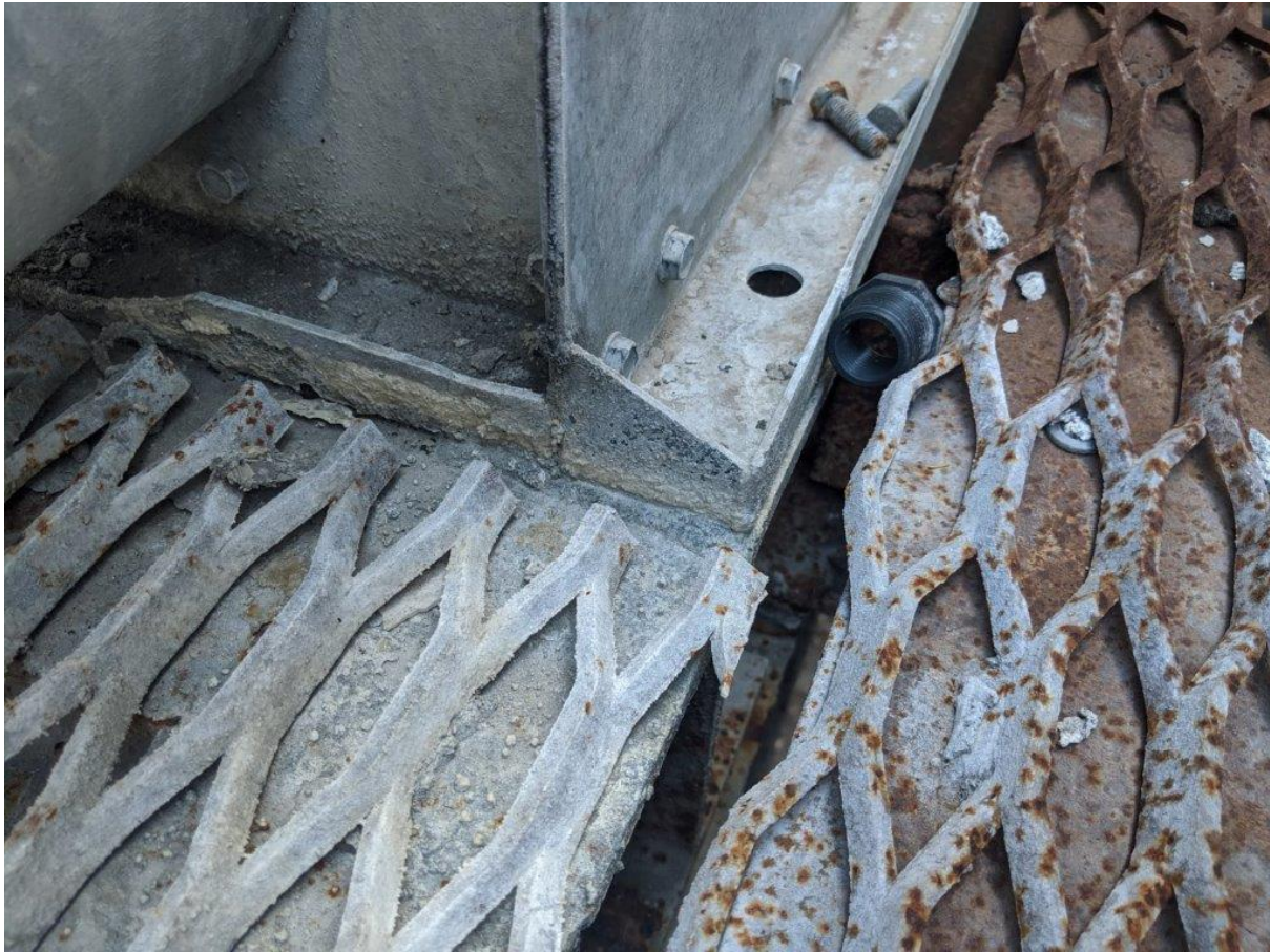
Caption 27. Condenser Anchorage (Typical)
