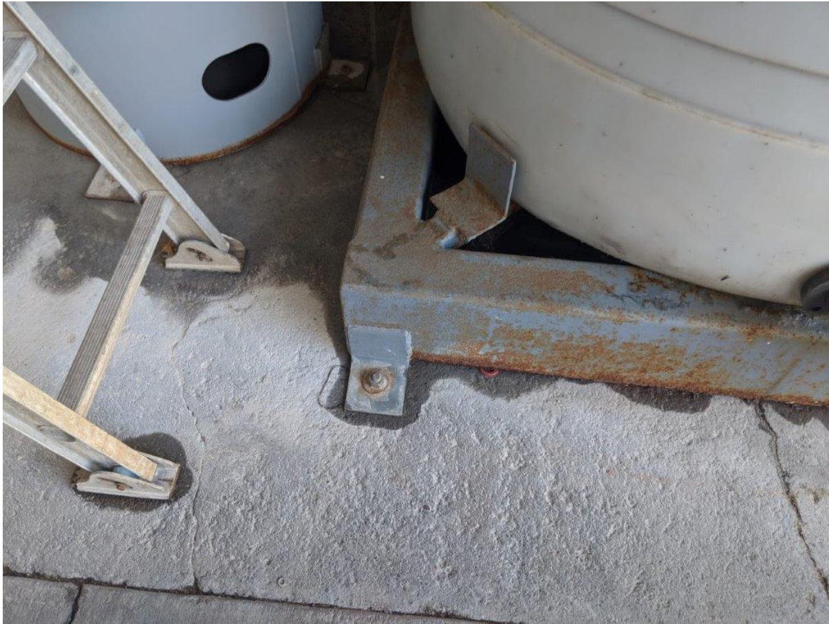
Caption 29. Glycol Chiller Skid Anchorage (Typical)
