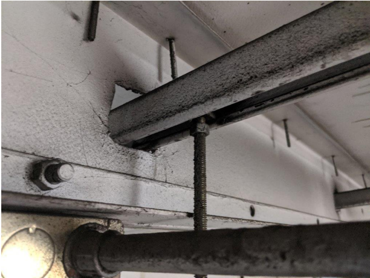
Caption 18. Evaporator EV1 Support Structure [ Action Item 3 ]
