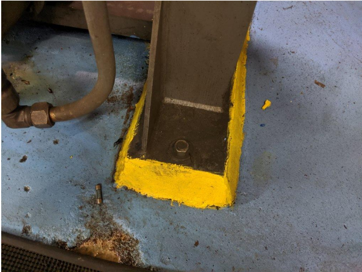
Caption 11. Compressor 1 Anchorage (Typical)
