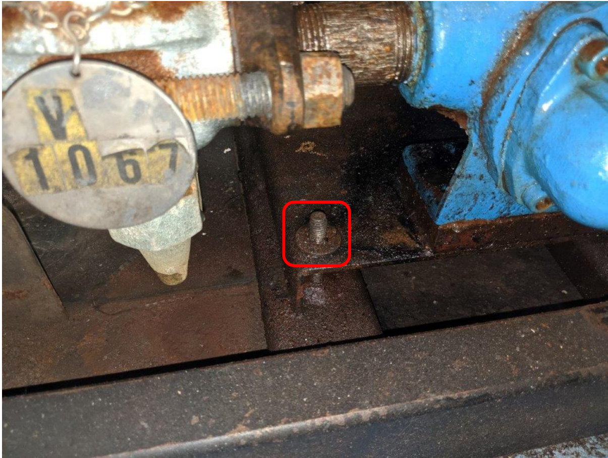
Caption 8. Liquid Transfer Pump Anchorage [ Action Item 2 ]
