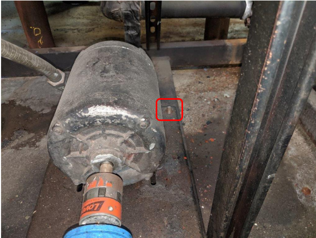
Caption 9. Liquid Transfer Pump Anchorage [ Action Item 2 ]
