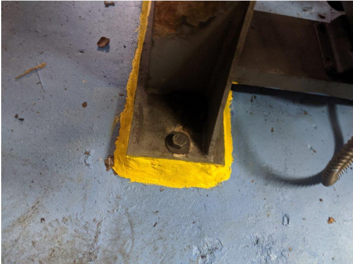
Caption 13. Compressor 2 Anchorage (Typical)
