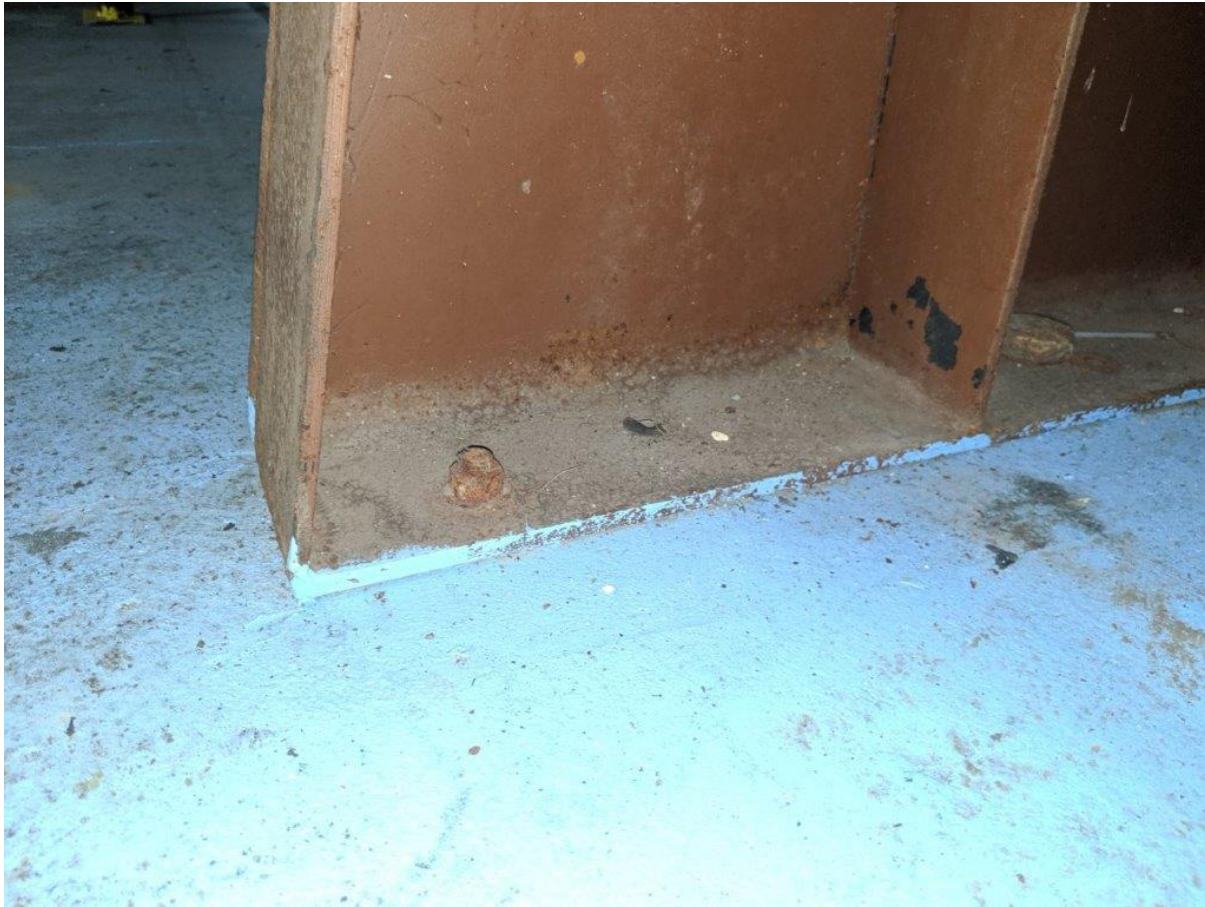
Caption 2. High Pressure Receiver Anchorage (Typical) [ Action Item 1 ]
